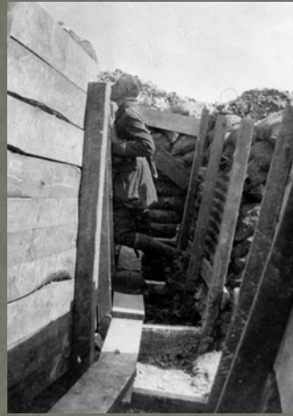
Reconstruction: "The centre sector was so demolished that a new trench line had to be dug in front and the three craters, which we named Cuthbert, Clarence, and Claude... had to be put into a state of defence..."
