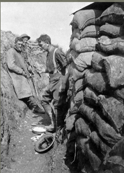
Toilet, Company Headquarters K1 Trench Arras: "what sort of sanitary arrangements, so very essential to health, could be made under conditions such as these? We used large buckets, which were emptied and disinfected every night, the contents being buried out on top by the sanitary squad consisting of two men per company acting under a corporal."
