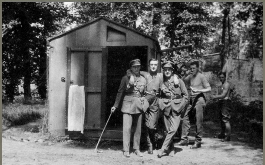
Agnez-les-Duisans rest billets (left and above), west of Arras: "Bathing facilities were also a very welcome and necessary feature of our existence, sheds having been erected under Corps arrangements and fitted with rows of hot water showers... clean underclothing was issued at the same time. The Quartermaster Sergeant brought up a clean pair of socks each night with the rations... we were indebted to the Ladies Committee which was indefatigably knitting for us away back in Birmingham."
